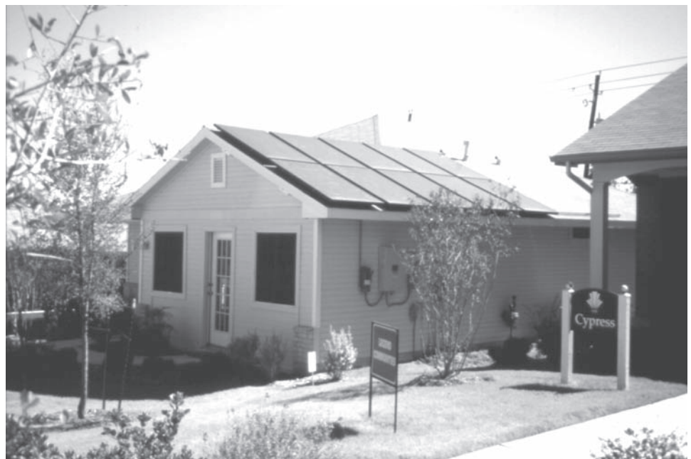
RESIDENTIAL PV SYSTEM The solar panels on the roof produce electricity that travels through wires to the distribution panel on the side of the home.
