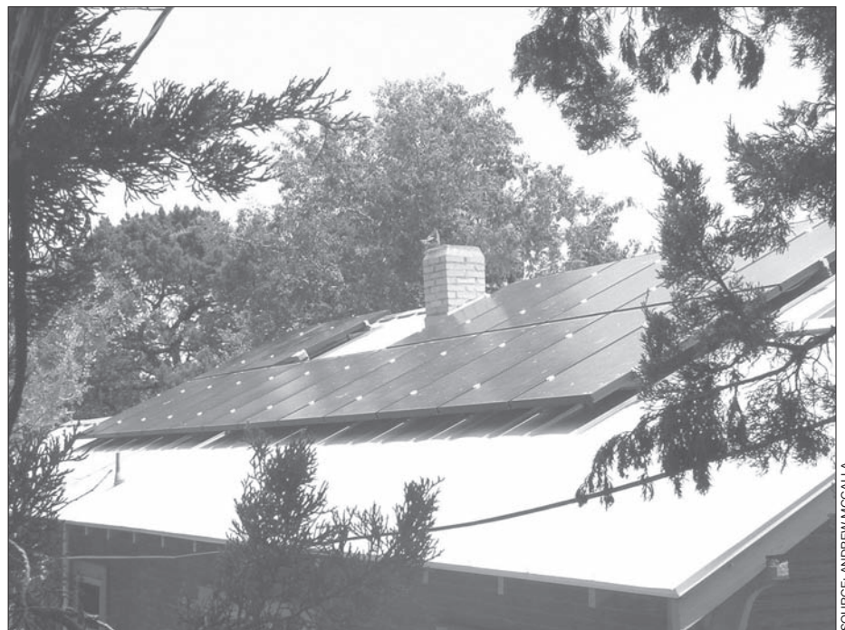
GRID-CONNECTED RESIDENTIAL PV More Austin homes are using solar electric systems tied to the utility for their power.
