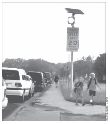
**SCHOOL CROSSING SIGNAL POWERED BY PV** Photovoltaics can provide small amounts of power that can be depended upon.
