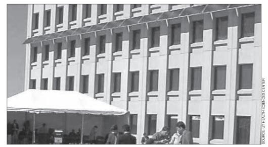
**BUILDING INTEGRATED PV PANELS** The University of Texas Health Science Center in Houston has a wall mounted PV awning to provide shade for windows below it as well as electricity.
