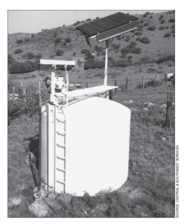
**USING THE SUN TO WATER LIVESTOCK** This PV system powers a small pump sitting on top of the water storage tank. During sunny weather, when cattle are most thirsty, PV watering systems work the best.
