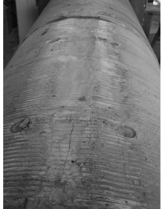
Fig. 25. Concrete core at northern side of the splice (see Figures 2 and 4).
